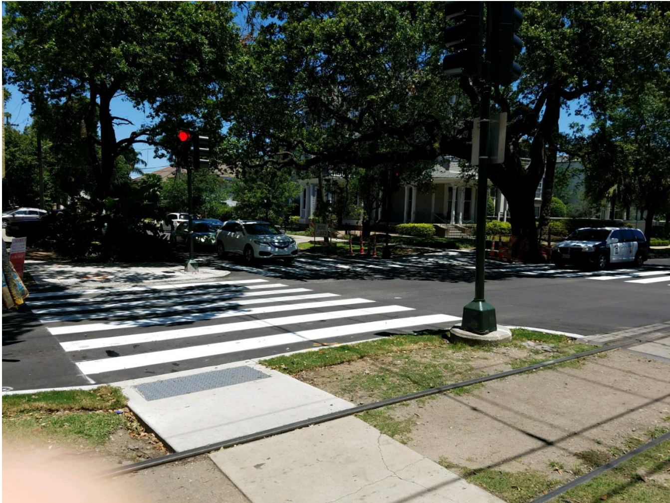
This portion of St. Charles Ave. was repaved and striped in 2017.
